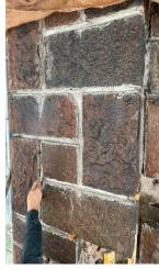
The first picture below shows the re-built parapet walls and second picture shows the condition with lifts 1 & 2 complete waiting for replacement stone. Once the stone arrives, it will be set using latex modified grout to close
